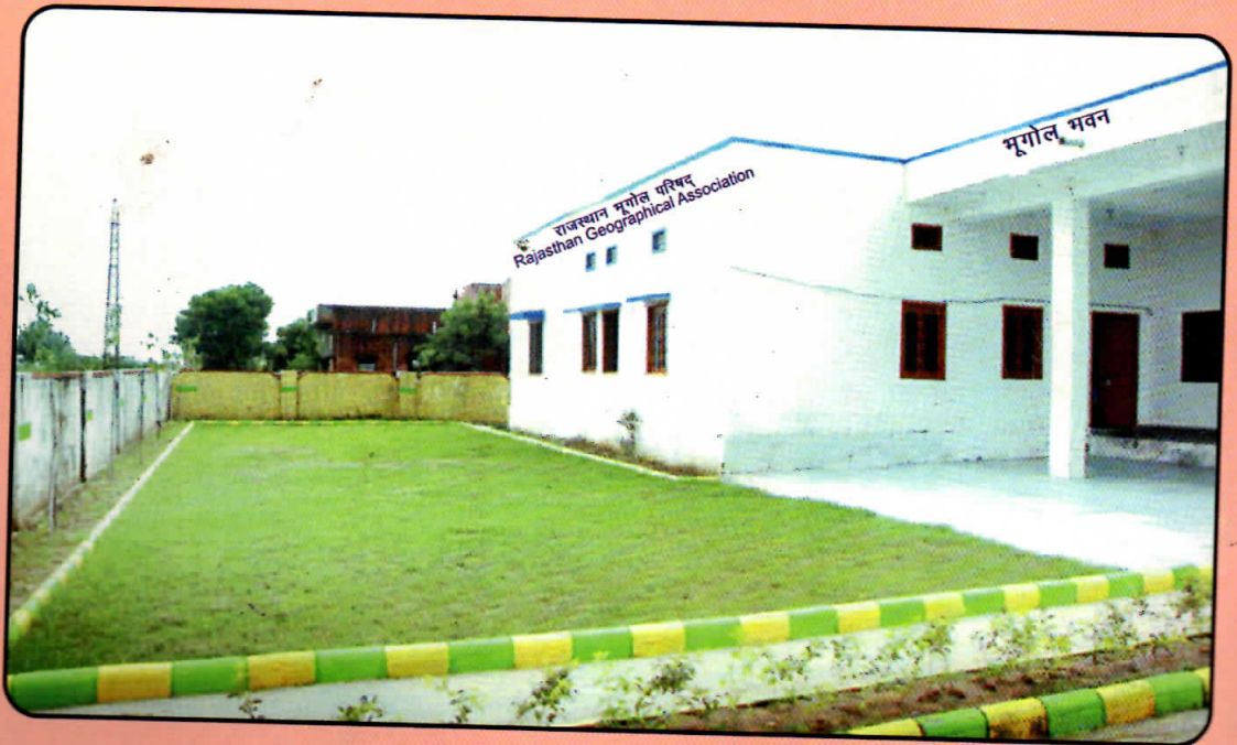
Bhoogol Bhawan Building Inner Front View
